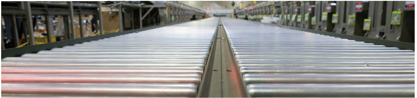
UPS MAIL INNOVATIONS PROCESSING FACILITY, FONTANA, CA
